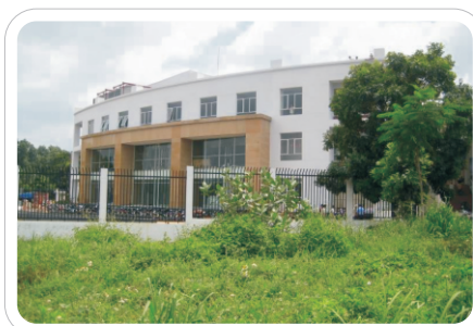
IGreen Data Center in Vietnam
